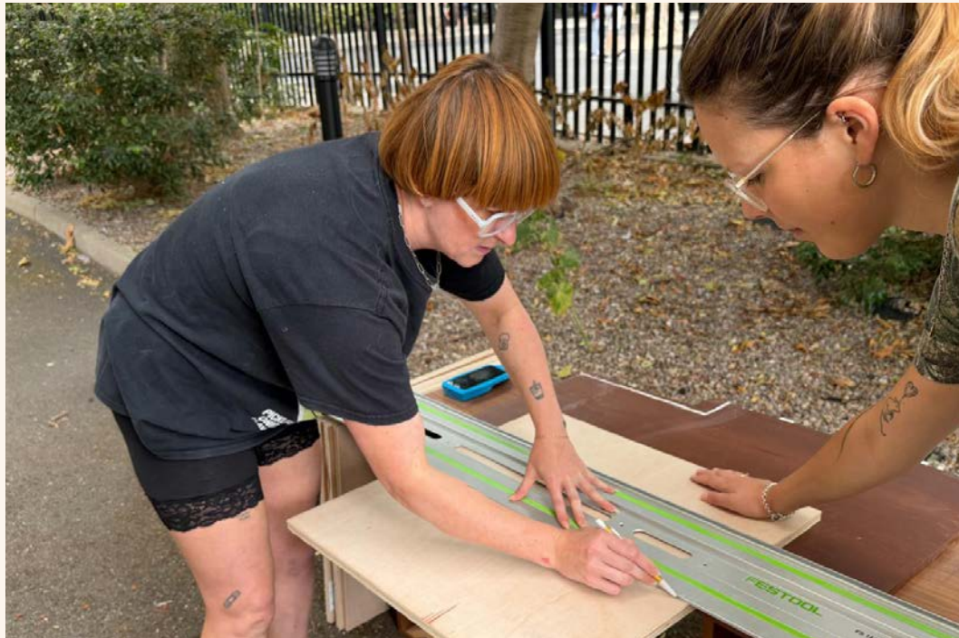
Zoë getting ready to cut bespoke floor pieces to fit around the trickier edges of the flat.
