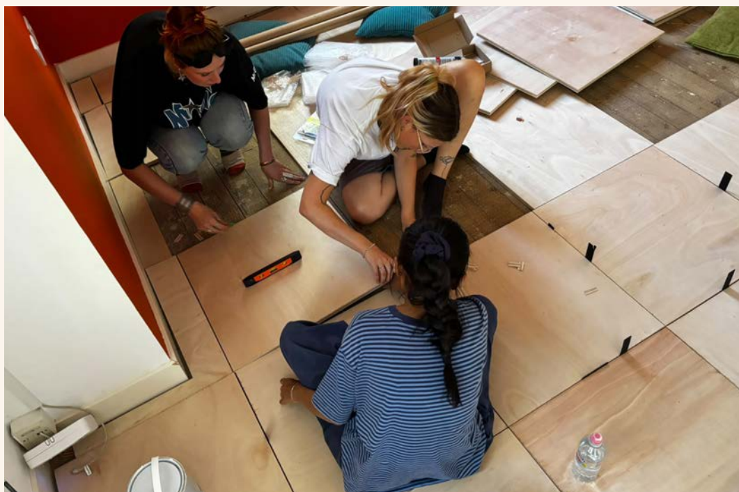
Abi, Bhairavi and Bry laying and levelling the floor, while Zoë makes custom shims just outside the Flat.
