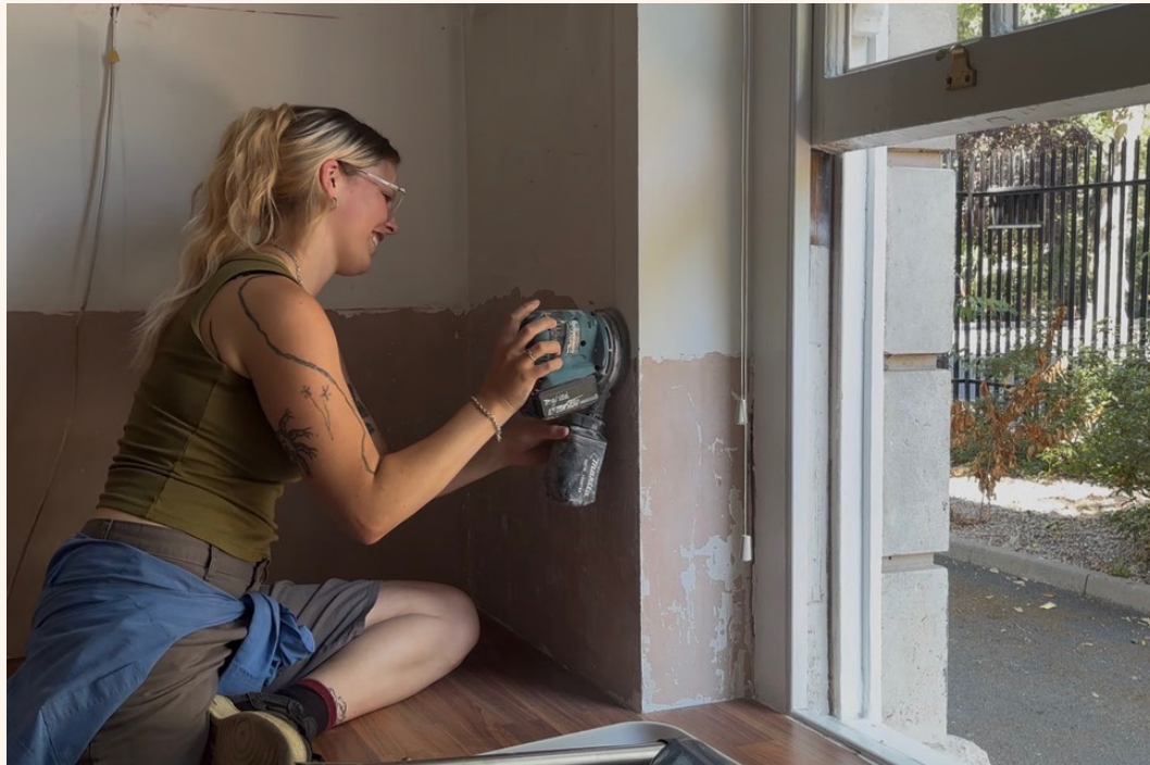
Abi sanding and smoothing the walls, getting them ready for their first coat of paint.
