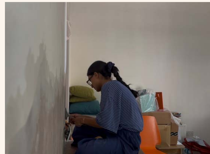
Bhairavi chiselling away the leftover grout from the kitchen tiles.
